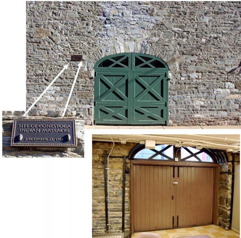
Portions of original County Jail foundation, and entry portal (exterior and interior) to former courtyard, location of 1763 massacre of Native Americans.
