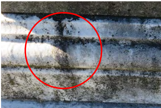
Stone #1 Rear: Cracking at Pin Locations
