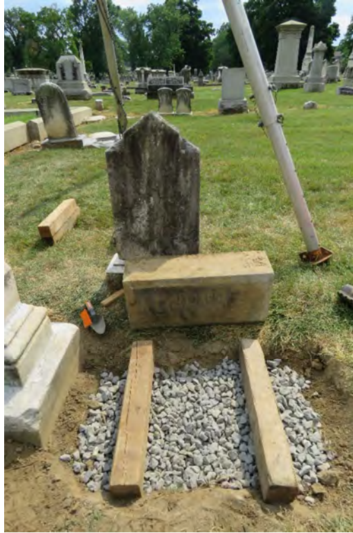
Stone #2 Die & Tier Unit and Base Moved with New Foundation Bed
