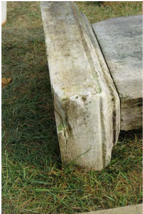
Closeup Views of Tier Corner Damage
