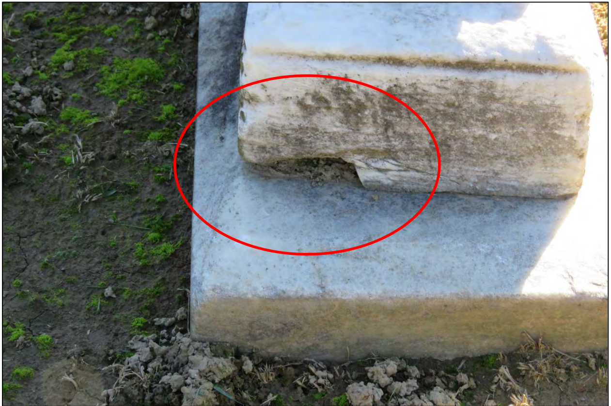
Stone #2: Tier – Left Side missing chip
