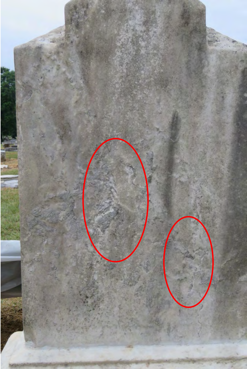
Stone #2: Flaking on Rear of Die
