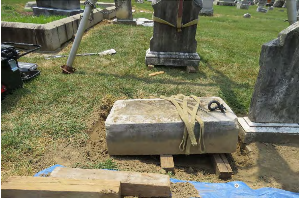
Stone # 1 Base Rigged and Lowered on to Shoring
