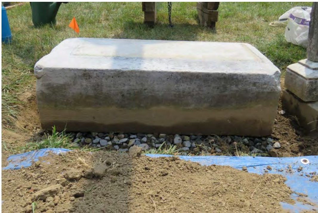
Stone #1 Base on a Bed of Drainage Rock
