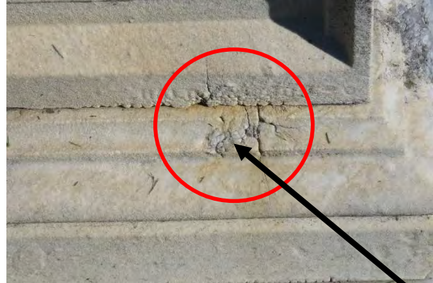
Stone #1 Front: Cracking at Pin Locations and quartz Inclusion
