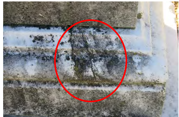
Stone #1 Rear: Cracking at Pin Locations
