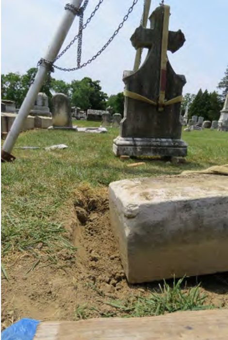
Stone #1 Die & Tier Removed and Placed on Shoring
