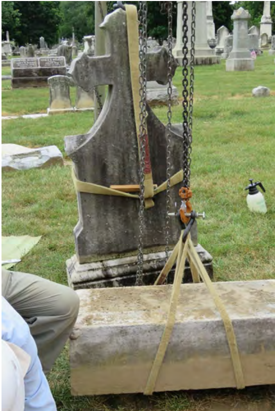
Stone #1 Base Raised and Base Foot Print Exposed
