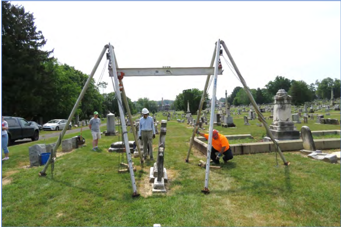
Gantry Completely Assembled
