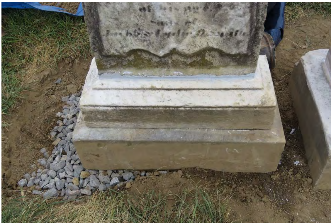
Stone #2 Reset on Bed of Drainage Rock
