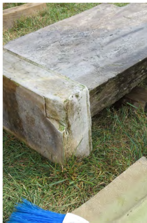
Closeup Views of Tier Corner Damage
